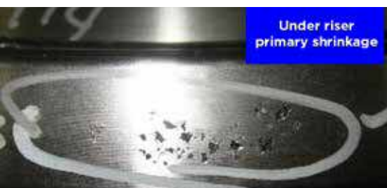
Figure 4. Porosity on machined face, under riser location.
